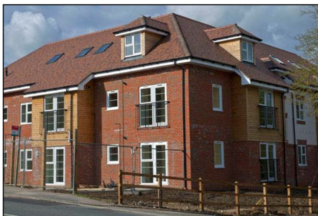
New affordable housing development at Vine Gardens
